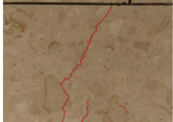
An example of tile cracks marked with high precision.
